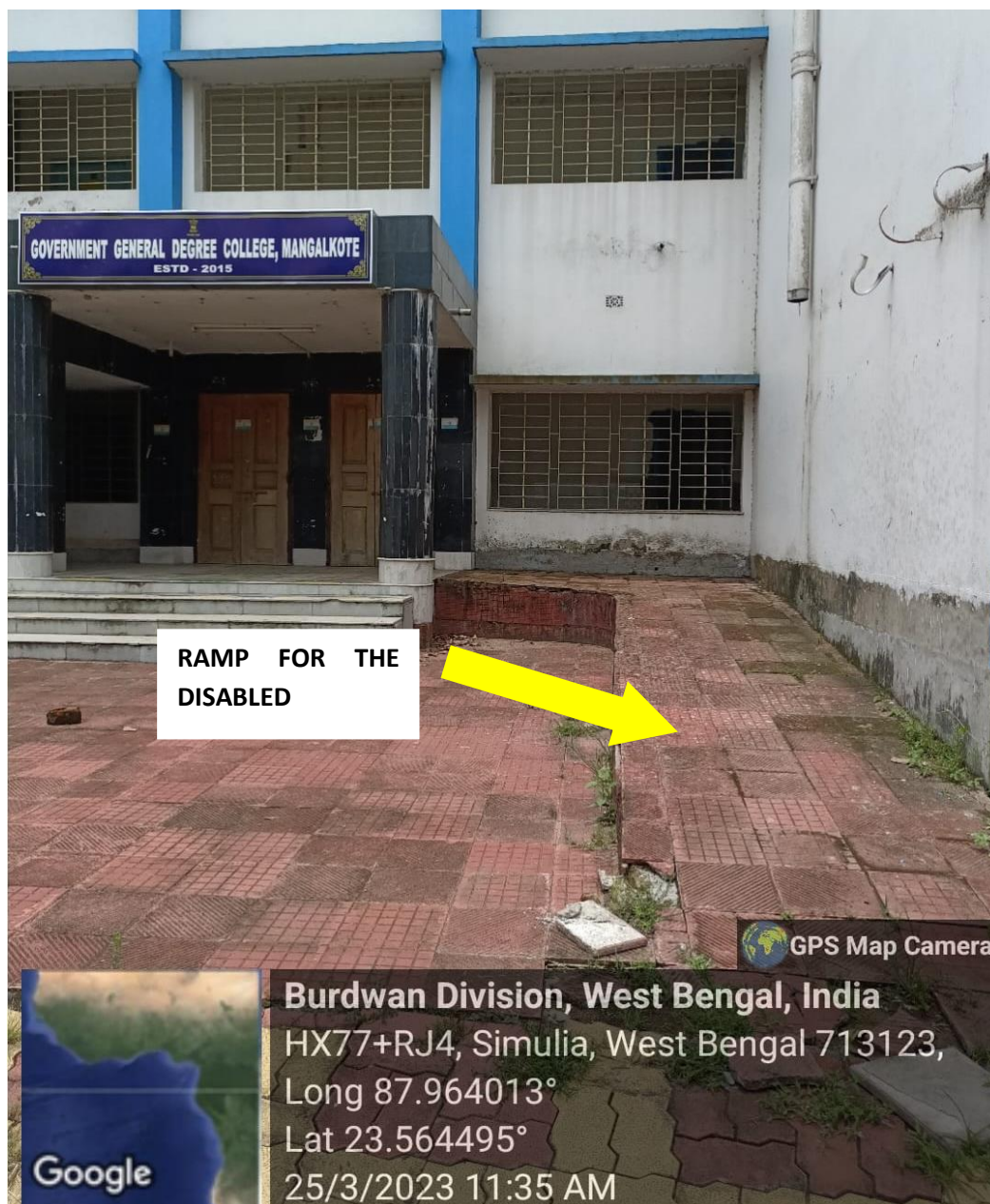
FIG.: RAMP FOR THE DISABLED STUDENTS
